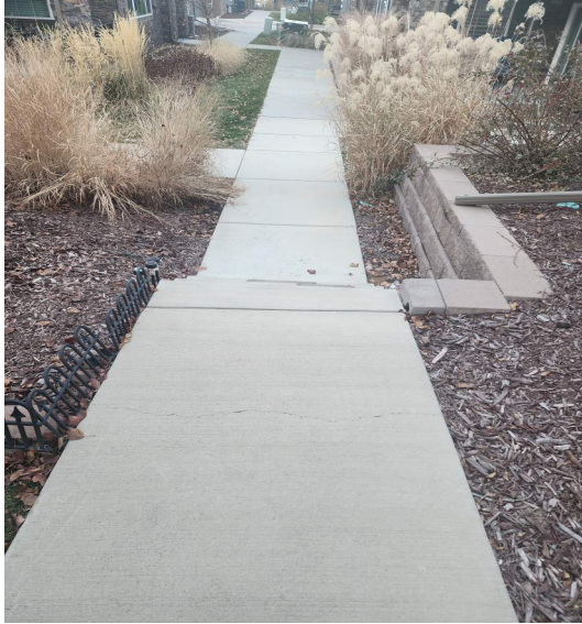
5. Cracked sidewalk
